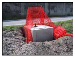
NOTE: the dimensions of the plinth are calculated on the coefficient of ground pressure, weight of the photovoltaic lamppost and windiness of the place. As it was set in the project the battery case has been inserted in a reinforced concrete structure.
