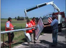
**STAGE 3:** installation of the cabling equipped lamppost with the help of a crane.
